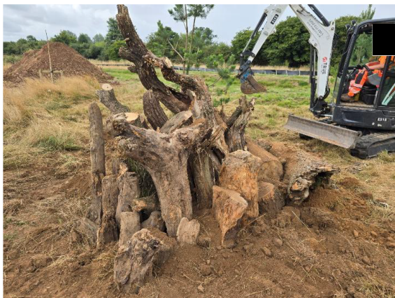
Image 22: Vertical log piles
